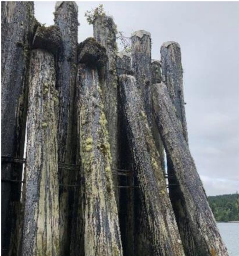
Photo 44 – North Mooring Dolphin
