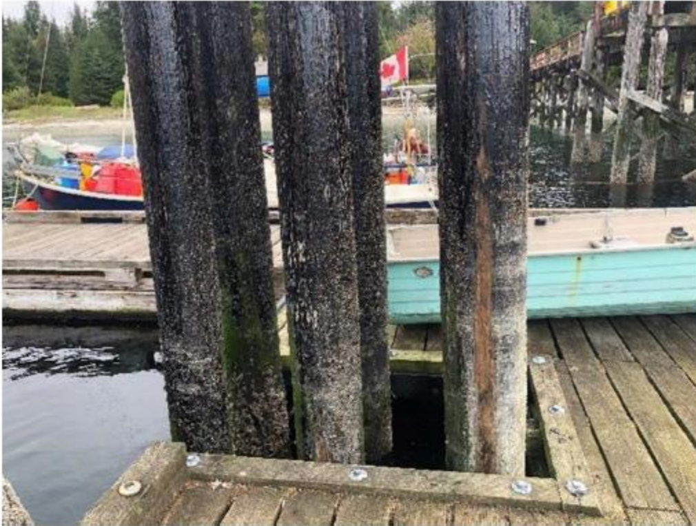
Photo 43 – Float A North Mooring Piles
