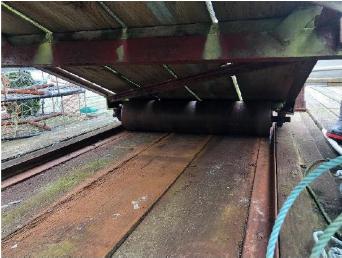
Photo 33 – Gangway Timber Slider Plate and Roller
