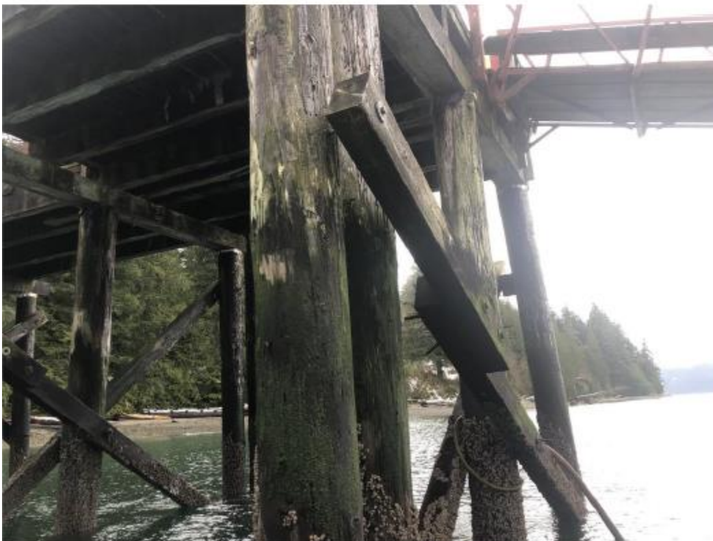
Photo 30 – Cross Bracing at Bent 15
