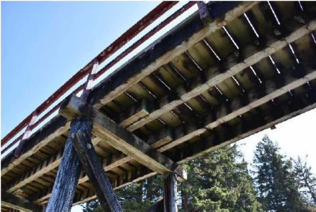
Photo 11 – Typical View of Timber Stringers
