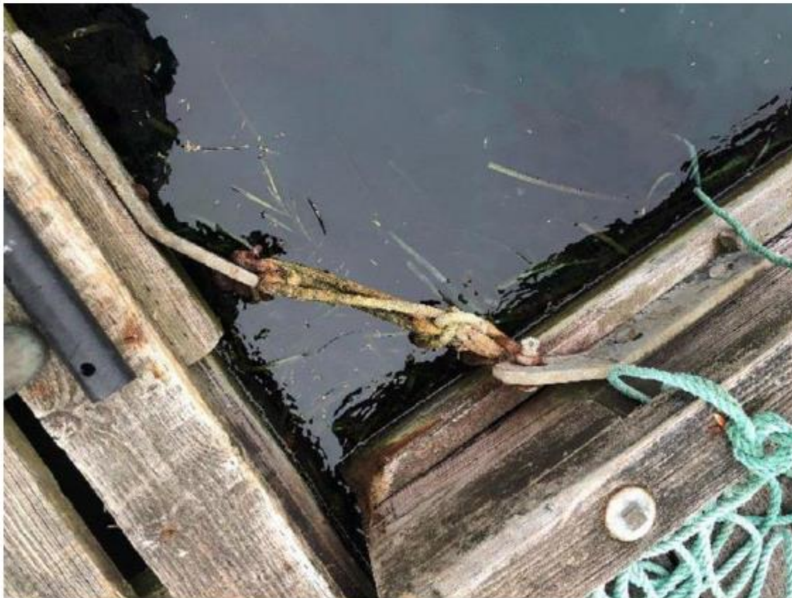
Photo 38 – Rope connection to Float B
