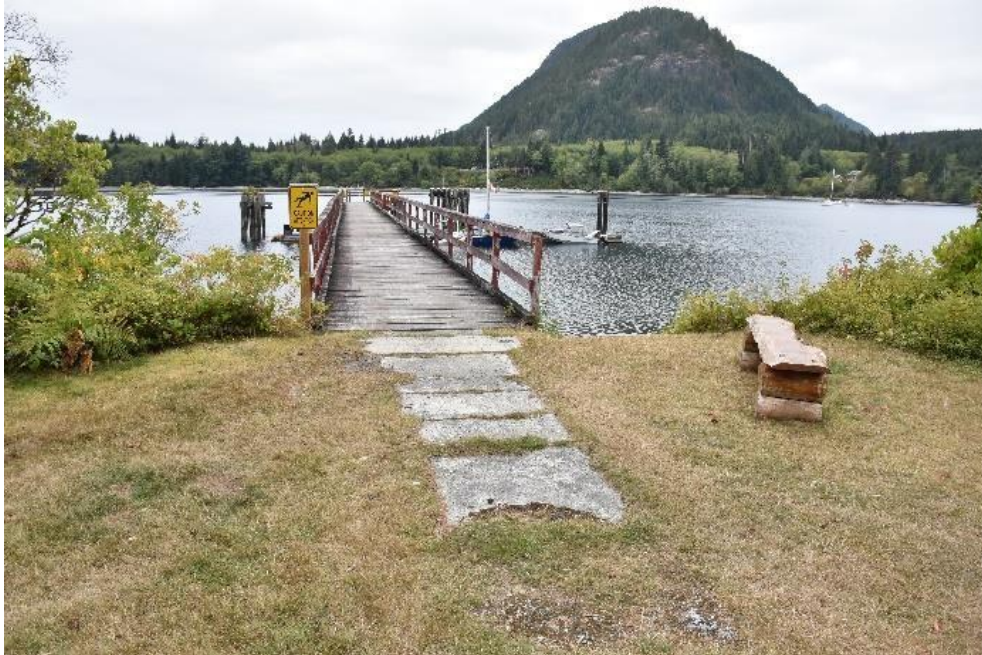
Photo 1 – Pier Approach Area
