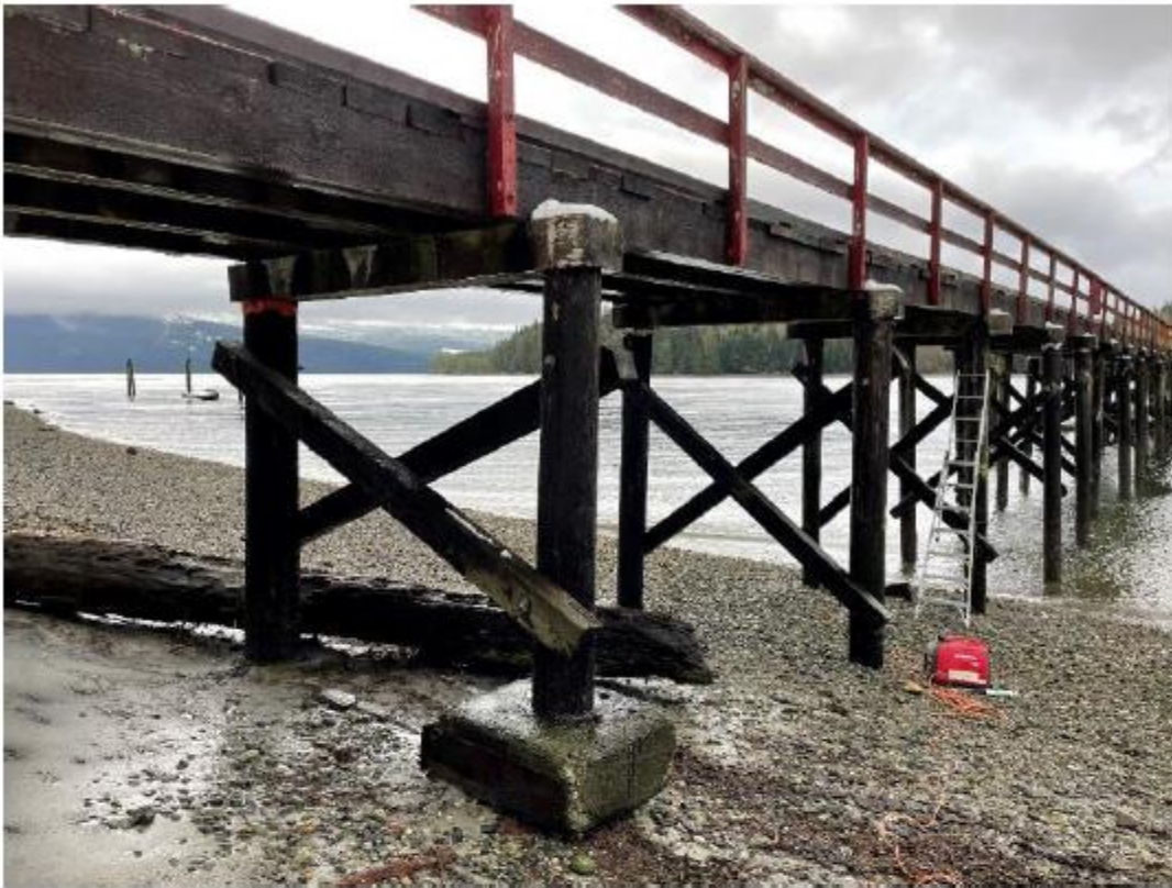
Photo 17 – Pile 4B concrete footing
