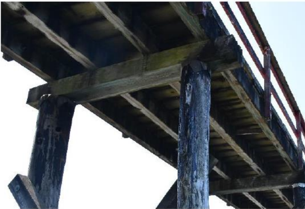
Photo 14 – Timber Pile Cap at Bent 12
