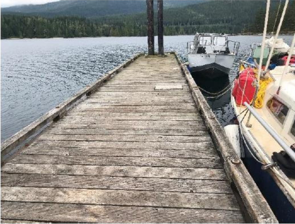
Photo 37 – General view of Float B
