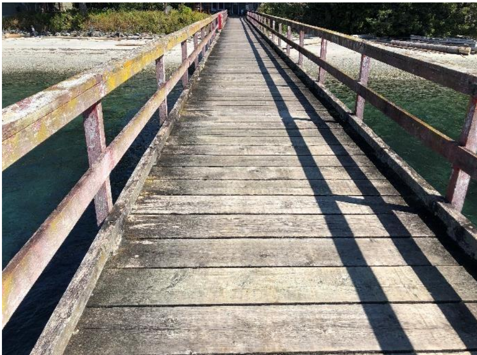
Photo 2 – Pier Structure Topsides
