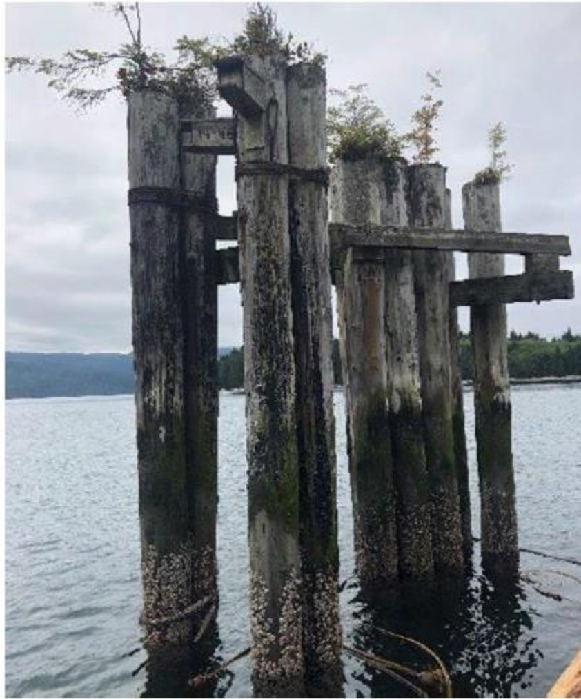
Photo 45 – South Mooring Dolphin
