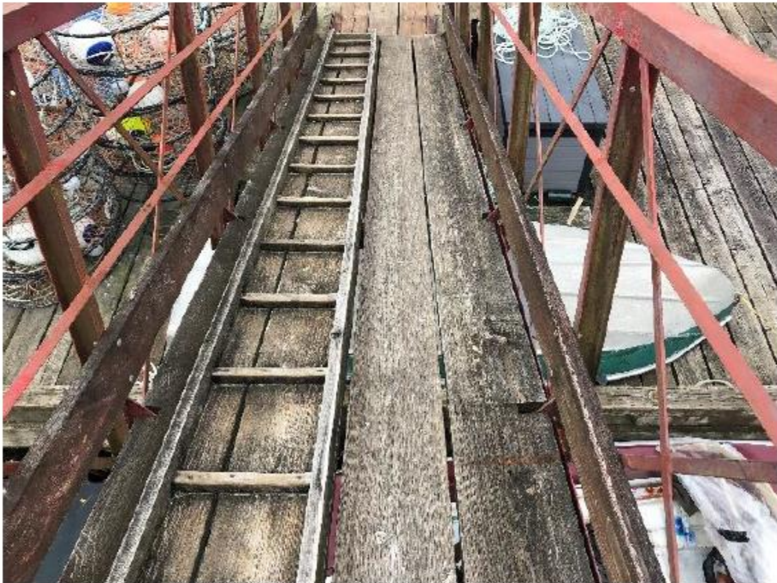
Photo 34 – Gangway Timber Deck Planks
