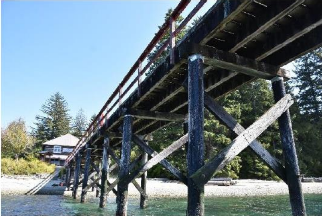
Photo 12 – General View of Timber Pile Cap Bents
