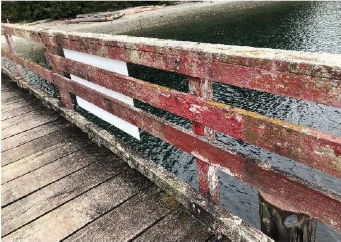
Photo 3 – Pier Structure Handrails
