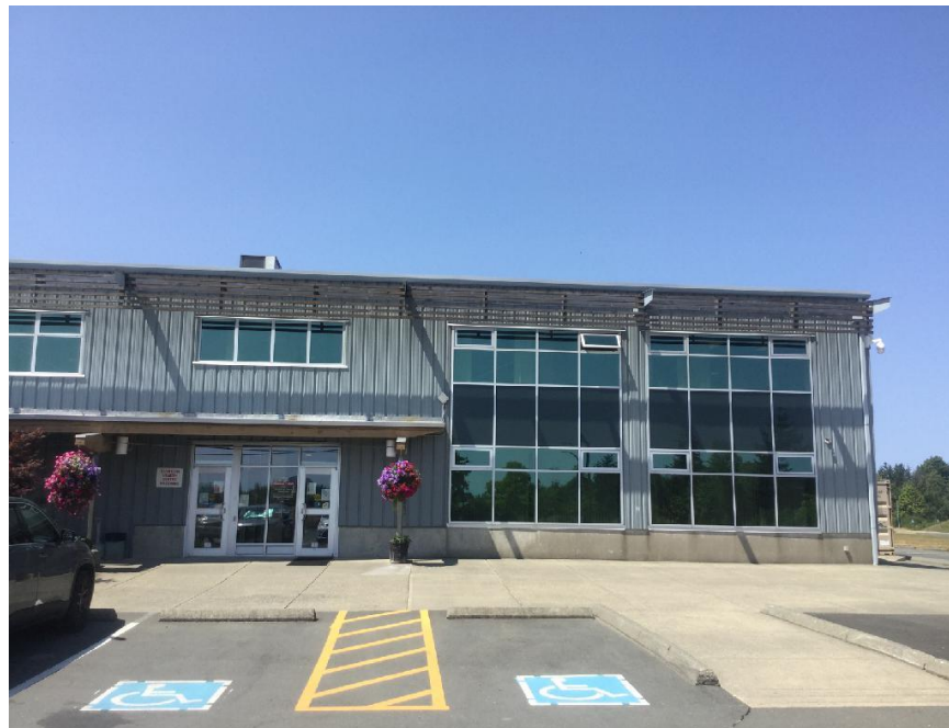
Figure 5: FireSmart compliance of the Quinsam Centre
