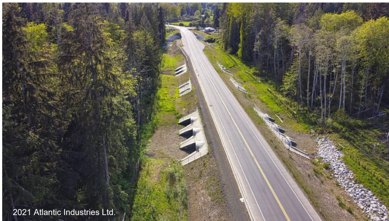
Figure 20: Percy Road Flood Relief Culverts, Atlantic Industries Ltd. 2021 ( www.ail.ca )
