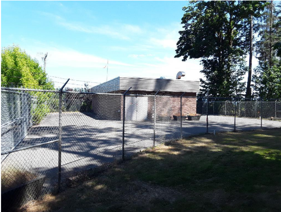
Figure 6: Oyster River Water Treatment Plant
