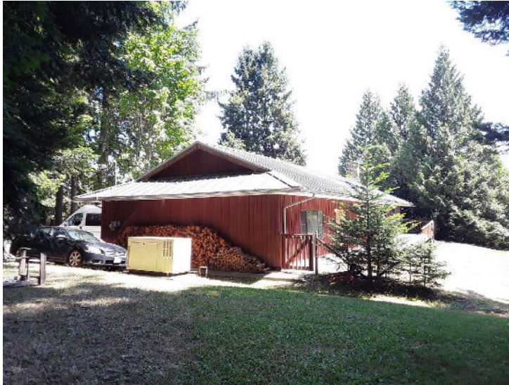
Figure 5: Example of combustible material (firewood) stored against a building in EA-D
